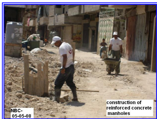
Construction of reinforced concrete manholes
