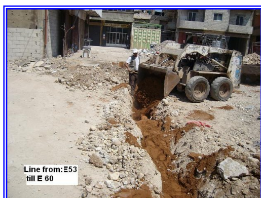
Installation of sewer lines
