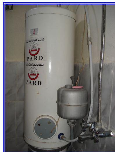
Photo of water heater installed
